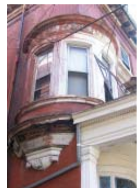
Masonry Ornate bay Window.
