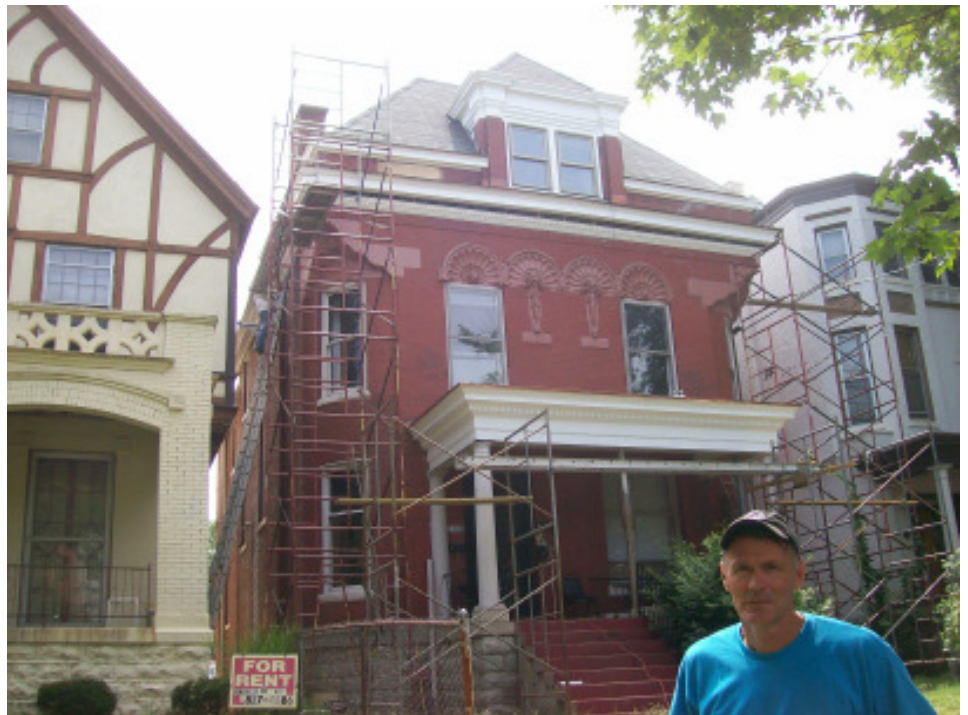
Substantial renovation underway at 1827 S. 3rd St. by Contractor Tom Boone.
