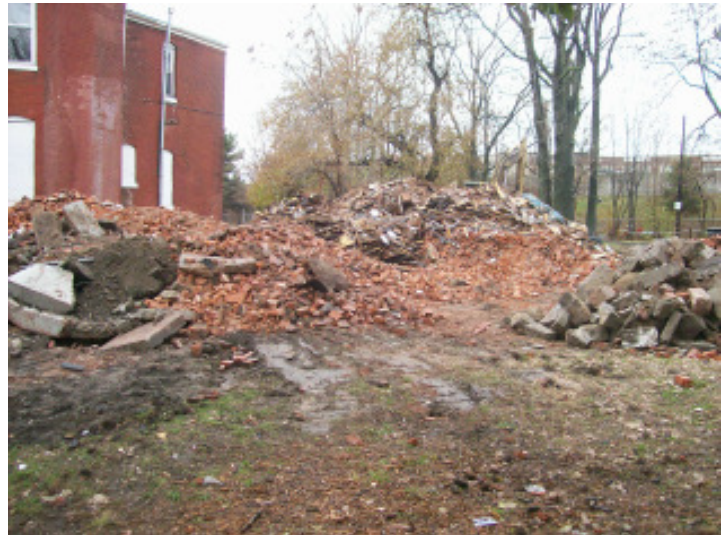
923 S. 1st St. demolished.
